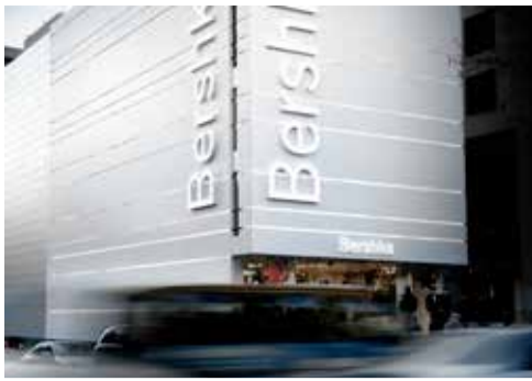
Bershka (Grupo Inditex) Location: Istanbul, Turkey Arquitect: Jordi Castel Designer: Jordi Veciana Project Manager: Jordi Castel Realization: Butech Building Technology
